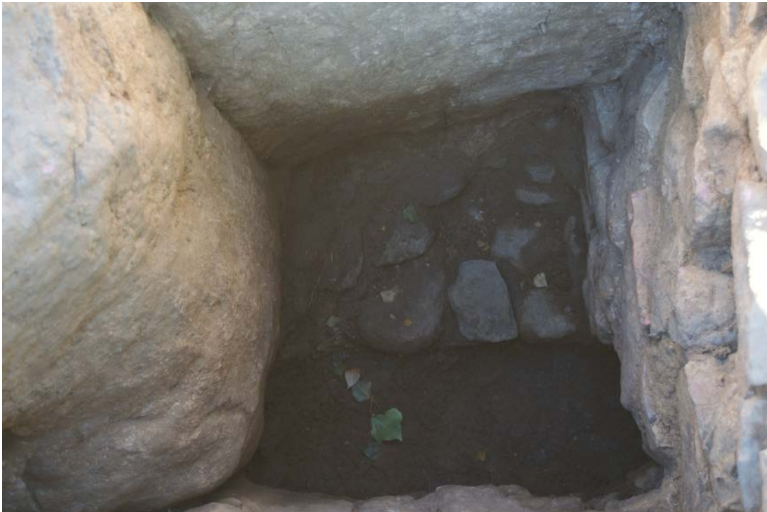
The floor of the catch basin.
