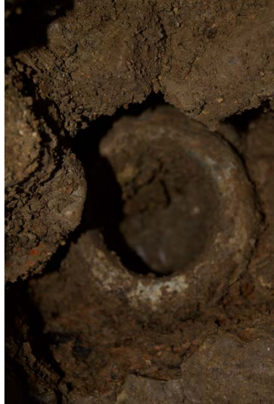
One of the lead pipes.
